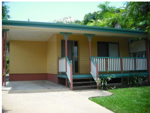
Figure SC6.2.3.23 Illustrates desirable outcome of a masonry constructed home with a "lightweight appearance"
